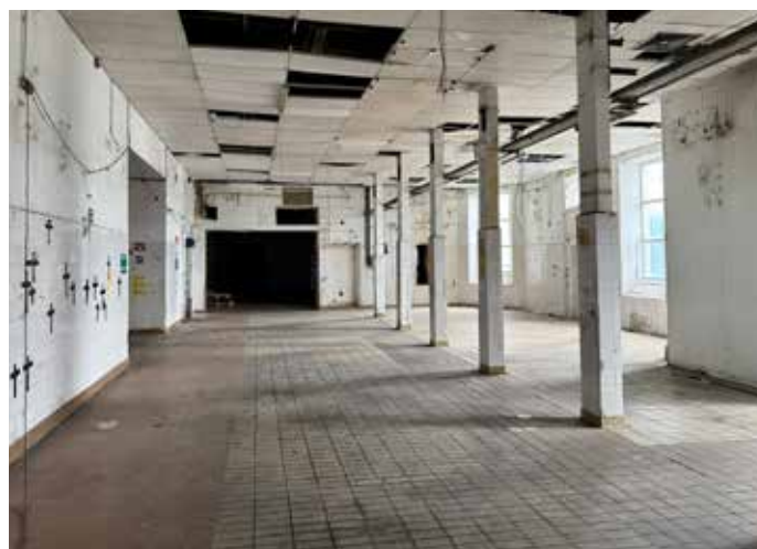
Fig.36 Extension c.1905, ground floor interior
