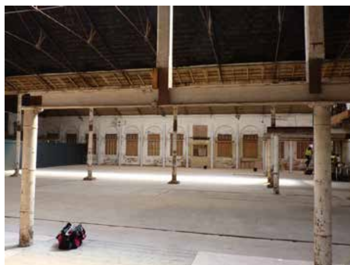
Fig.121 The dyehouse at Ditherington Flax Mill
