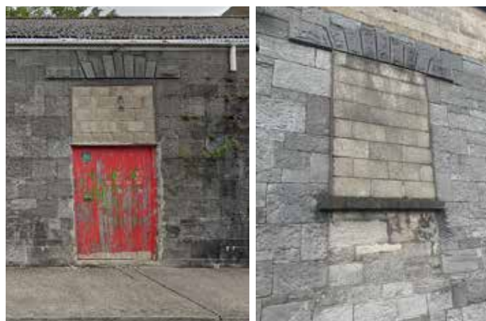
Fig.61 Adjusted window opening - shop entrance and reduced height
