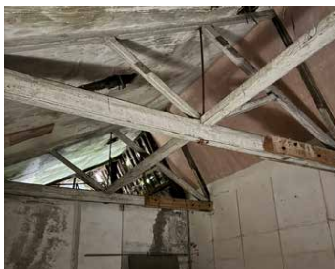
Fig.58 Roof structure of the long building
