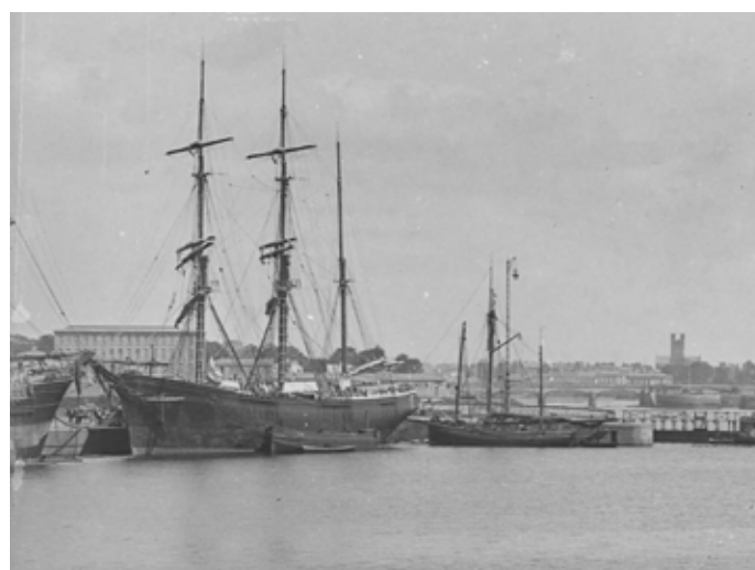
Fig.1 View from across the dock, 1890
