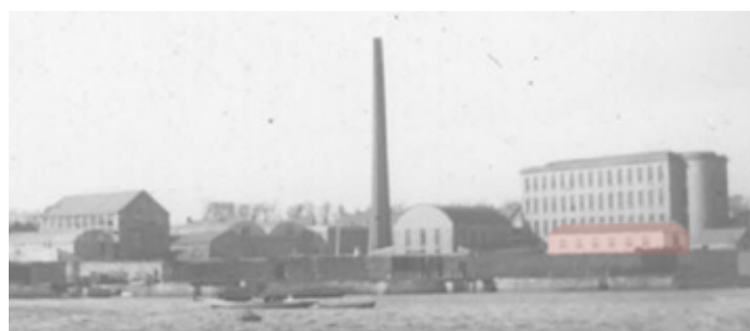
Fig.63 Photo of the site c.1900 - building highlighted
