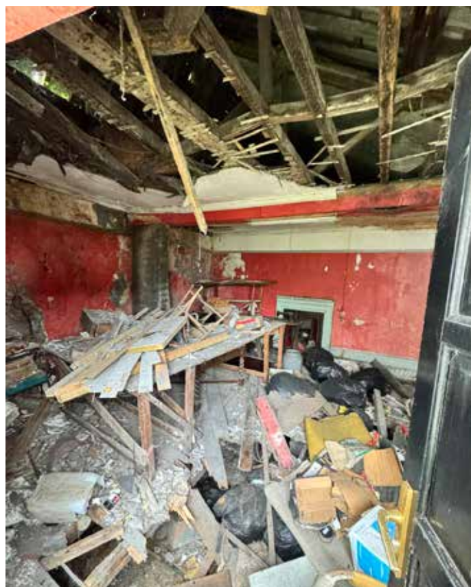
Fig.60 West room of the long building
