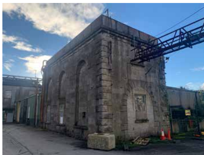
Fig.54 Water Tank building from ground level
