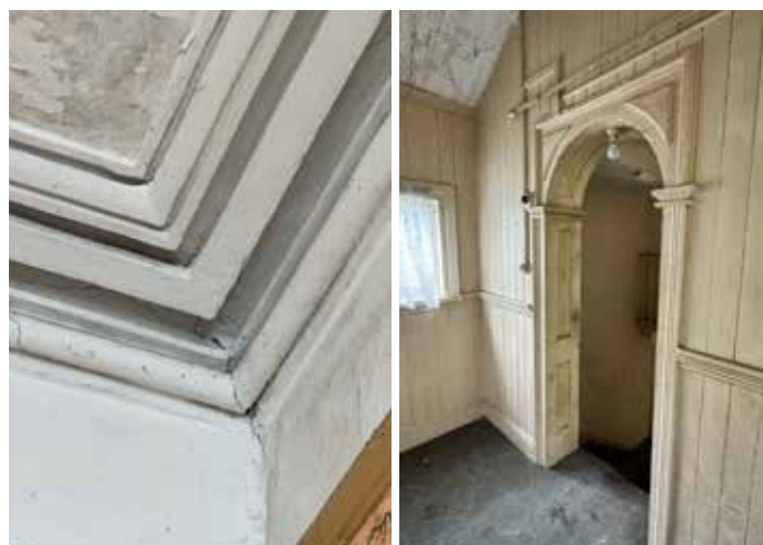
Fig.78 First floor cornice and decorative timber arch between stair and rear bathroom
