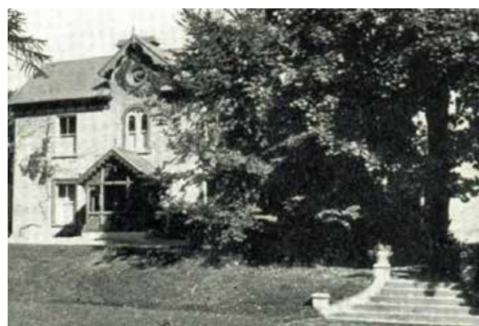
Fig.89 Fernbank House c.1930
