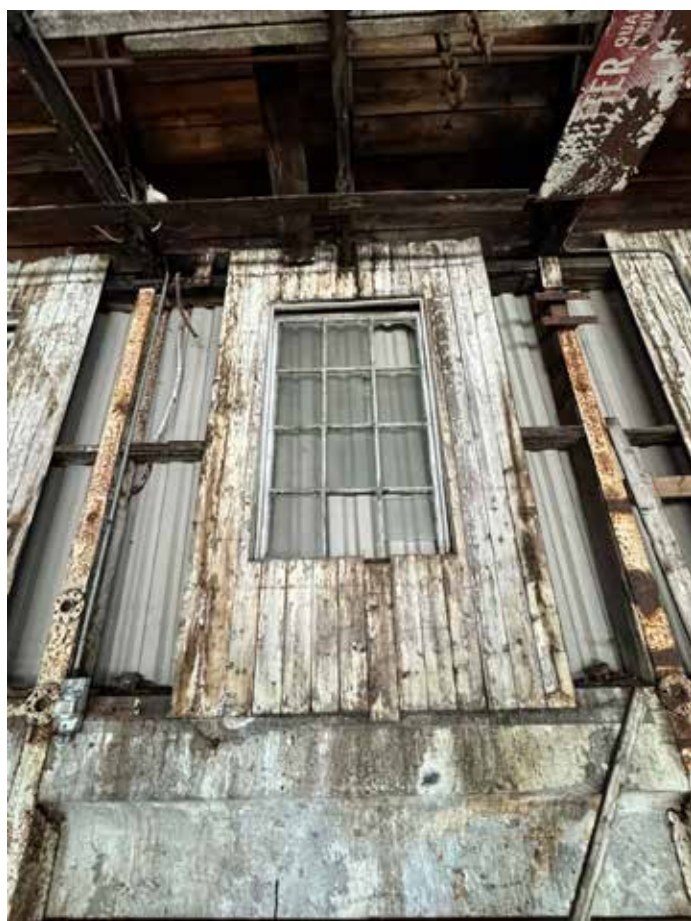
Fig.65 Photo of the workshop 12 pane window and timber boarded wall
