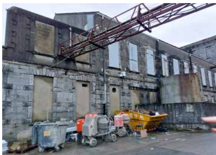
Fig.23 Junction between Weaving Mill phases with 1950s first floor over
