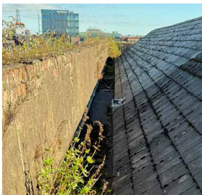
Fig.13 View along the north parapet.
