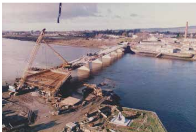
Fig.112 Construction of Shannon Bridge, 1986
