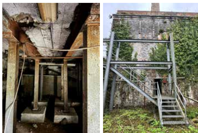
Fig.55 Water Tank building
