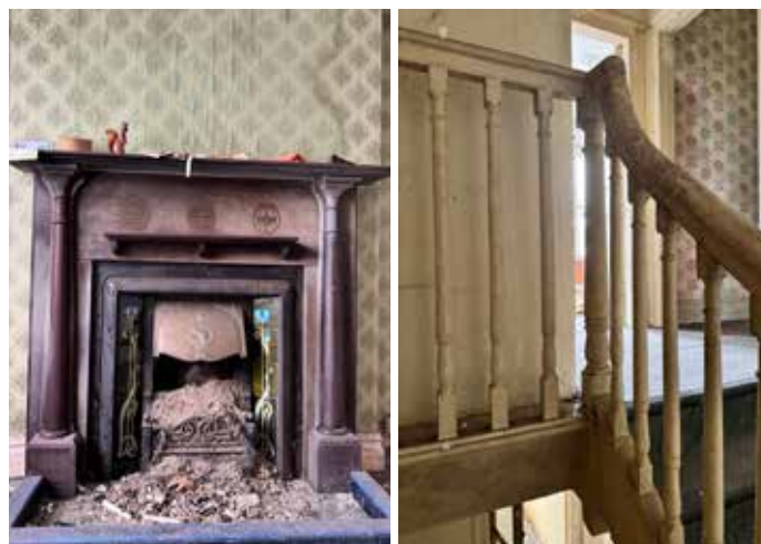
Fig.77 Fireplace with mantel and stair balustrade
