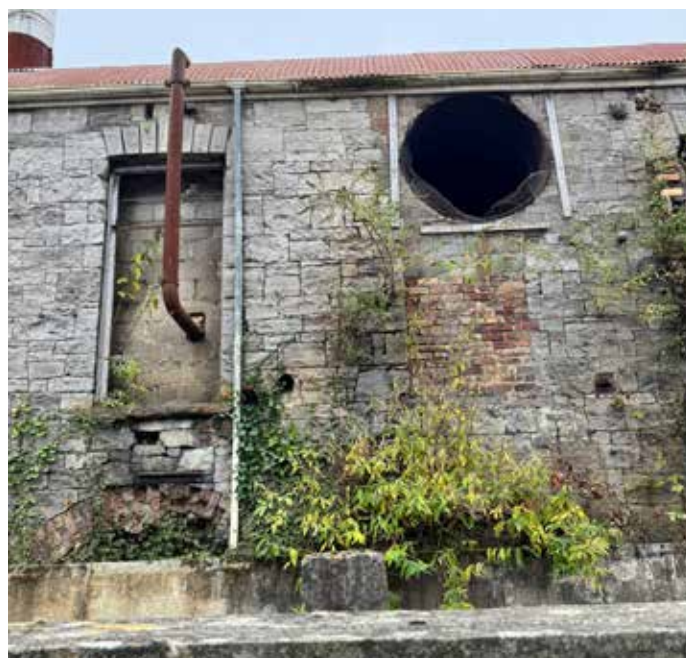
Fig.51 Space between the boiler house and chimney
