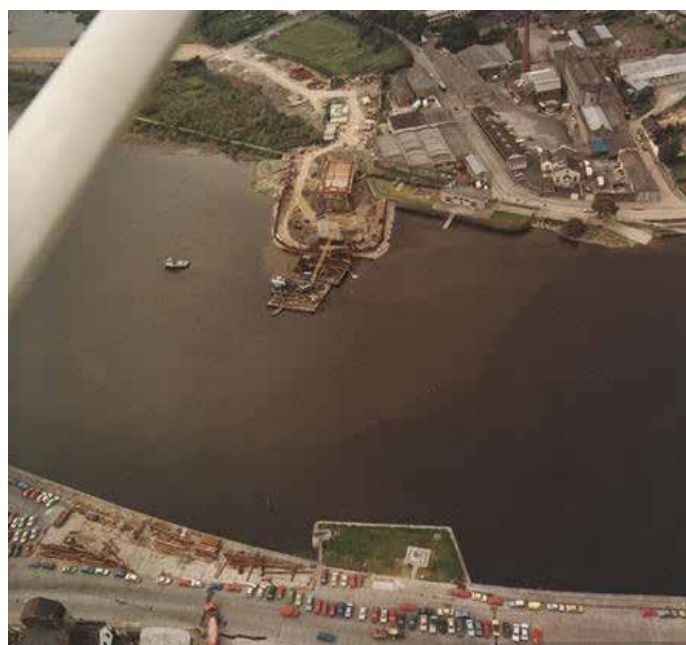
Fig.143 Construction of Shannon Bridge, 1985
