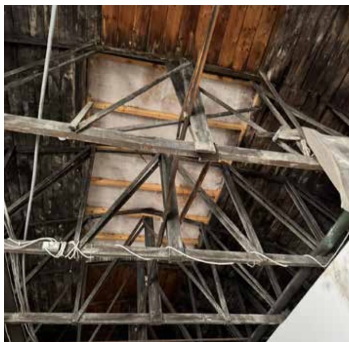
Fig.67 Photo of the workshop roof, lattice truss and vent opening
