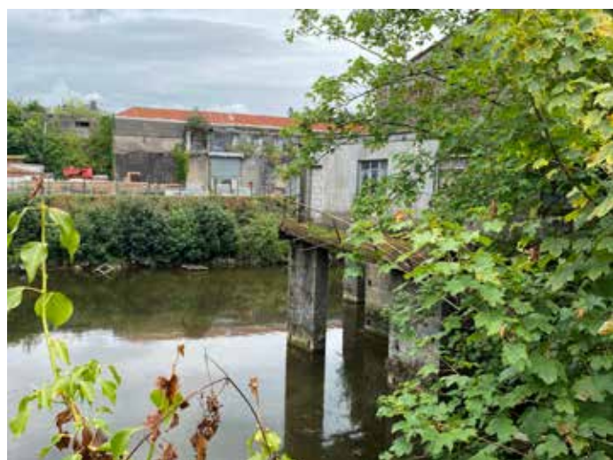
Fig.84 View over the reservoir looking north
