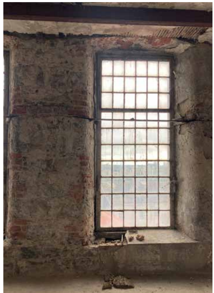
Fig.12 Window bay with iron band and jacking of masonry
