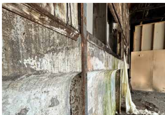
Fig.68 Photo of the corniced plinth and steel posts
