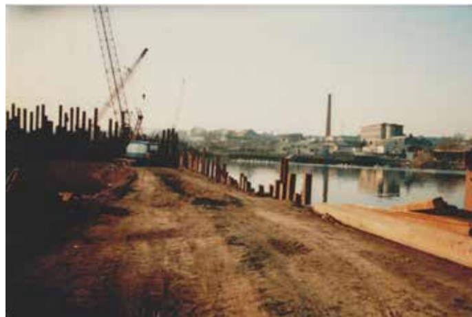
Fig.142 Construction of Shannon Bridge, 1985
