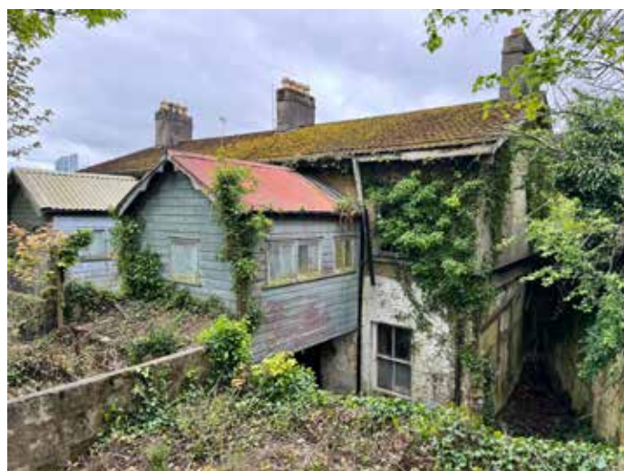
Fig.75 House - rear elevation
