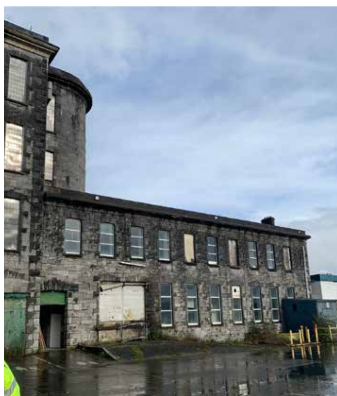
Fig.37 Extension c.1905, elevation onto the mill yard
