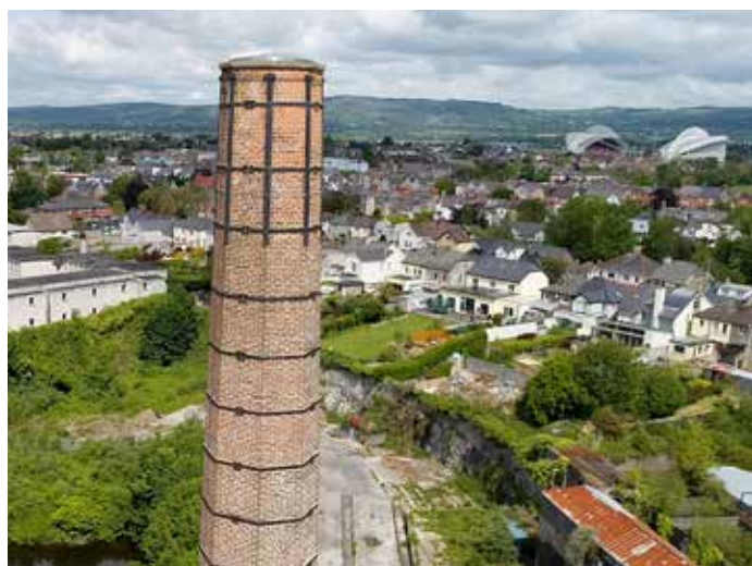
Fig.50 Brick Chimney 1852, with bands and modern capping
