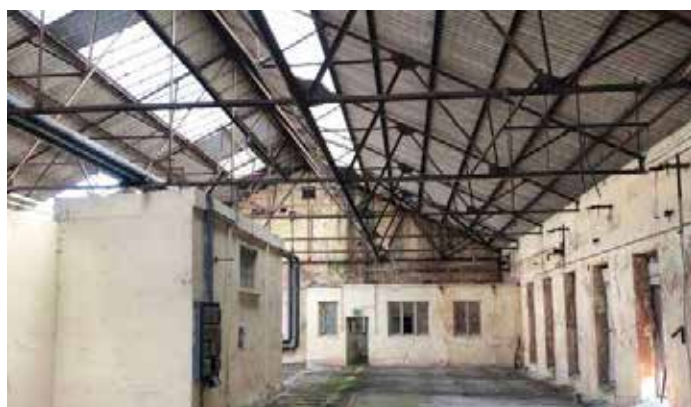
Fig.22 First floor of the Milk Separating Room. Formerly phase one of the Weaving Mill. 1951 roof structure with asbestos sheet covering.
